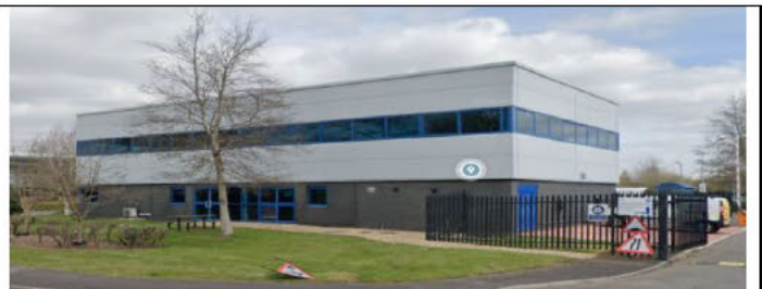
2 storey office Block
