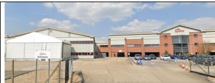
Warehouse with offices
