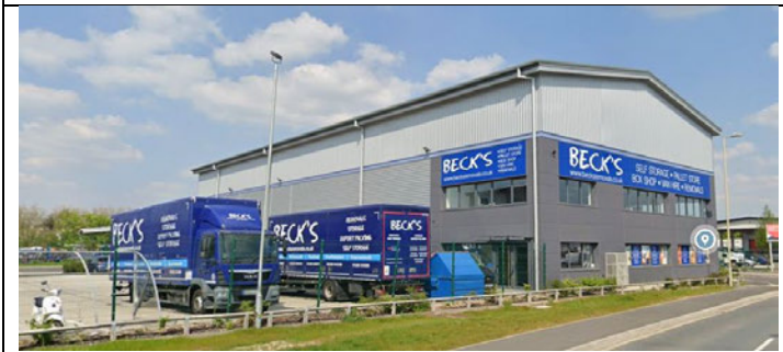
Warehouse with ancillary offices - Built in 2019
